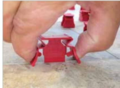
SeamClip works by interlocking the tiles, creating a single flat-slab surface while the setting material is curing. The interlocking design reduces or eliminates settling from shrinkage, and minimizes the possibility of warping. The result is a lippage-free mirror surface that reduces the need to re-lift tiles to add more mud, or to shim tiles. [www.pearlabrative.com](http://www.pearlabrative.com)
